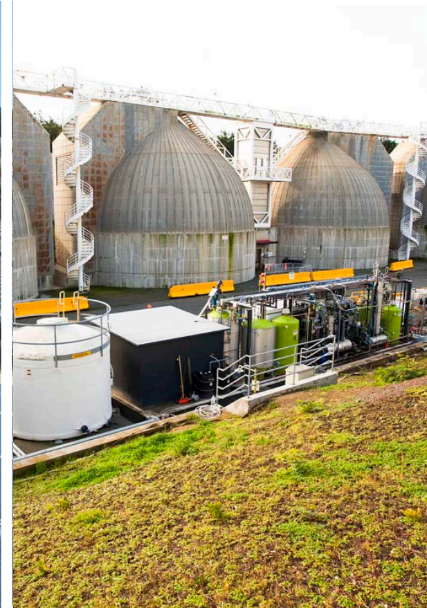
Oceanside Treatment Plant
