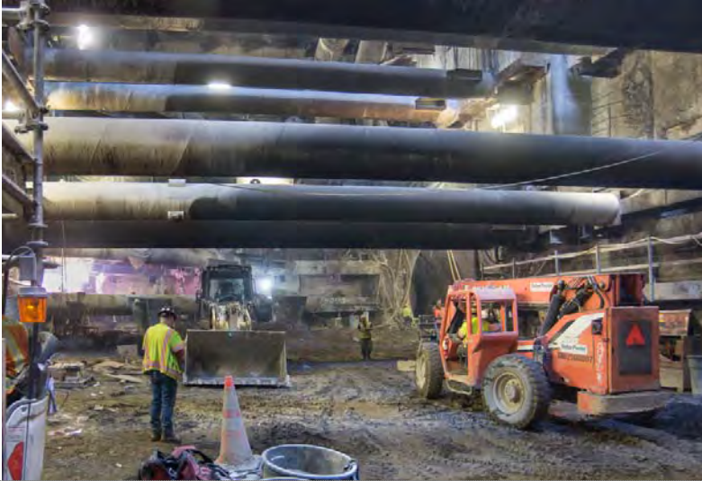
1 An initial level of excavation is conducted and equipment reorganized
