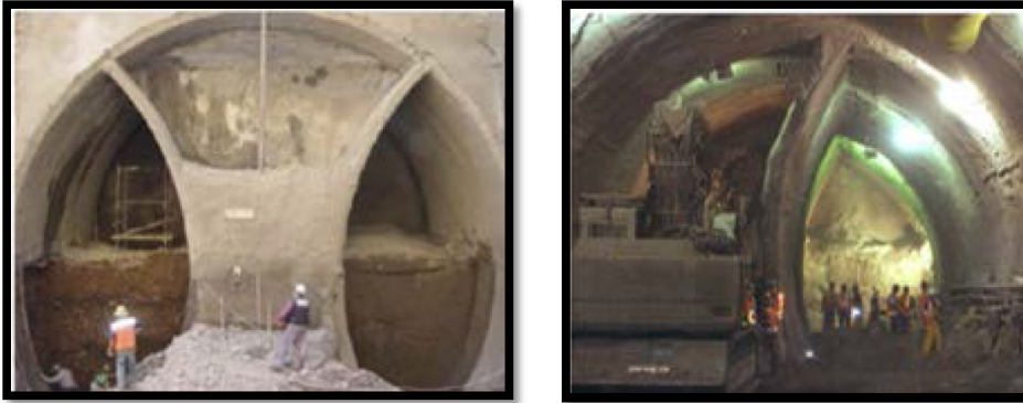
Figure 4.2.13 & 14 Excavations by Sequential Excavation Method (SEM)
