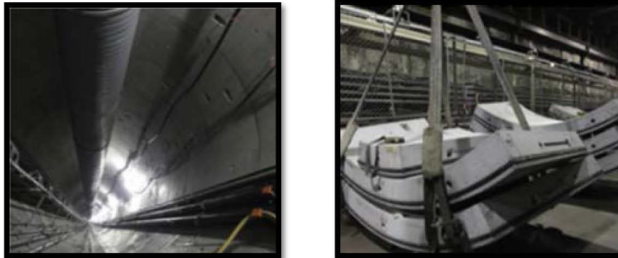
Figure 4.2.7 & 8: T Third Phase 2 – Lined tunnel and precast segments
