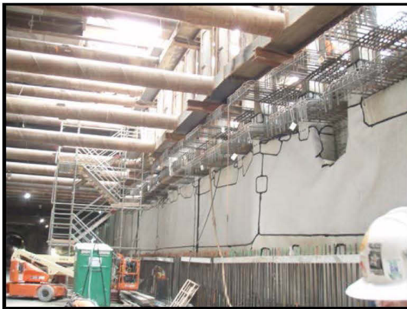
Figure 4.2.22: Station Box Excavation and Support
