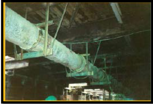
Figure 4.2.23: Major utility pipe supported off street decking
