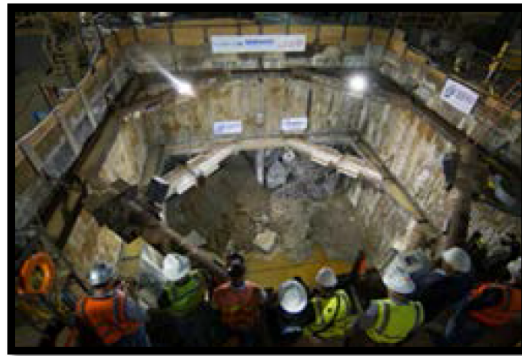
Figure 4.2.11: TBM retrieval shaft at Pagoda Site
